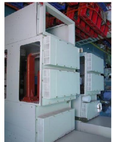
Cooling duct for high current rating
